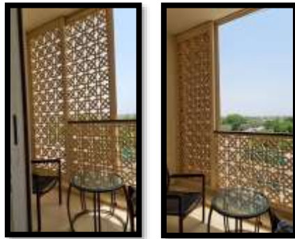
Figure 8. Modern design of mashrabia in the form of sliding screen used at the balcony of Barceló resort Mussanah, Oman.
