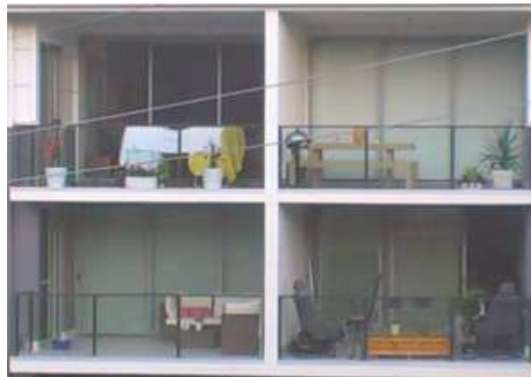
Figure 7. Glass balustrade reduces the visual privacy, especially at night when curtains are put aside. Source: Kennedy et al., 2015
