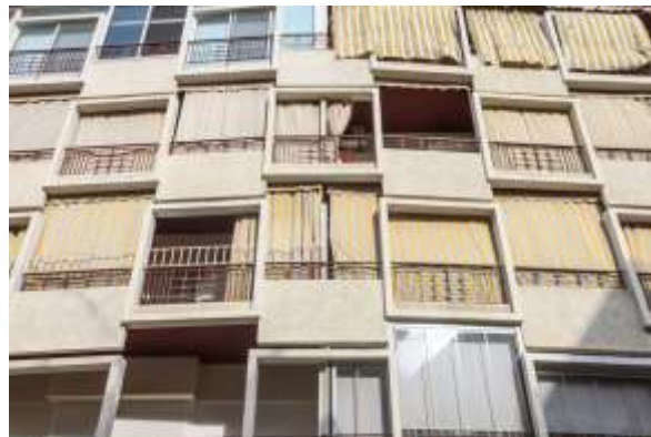
Figure 9. Curtains to control the level of privacy, interaction, and sun exposure level on their balconies in Beirut, Lebanon
