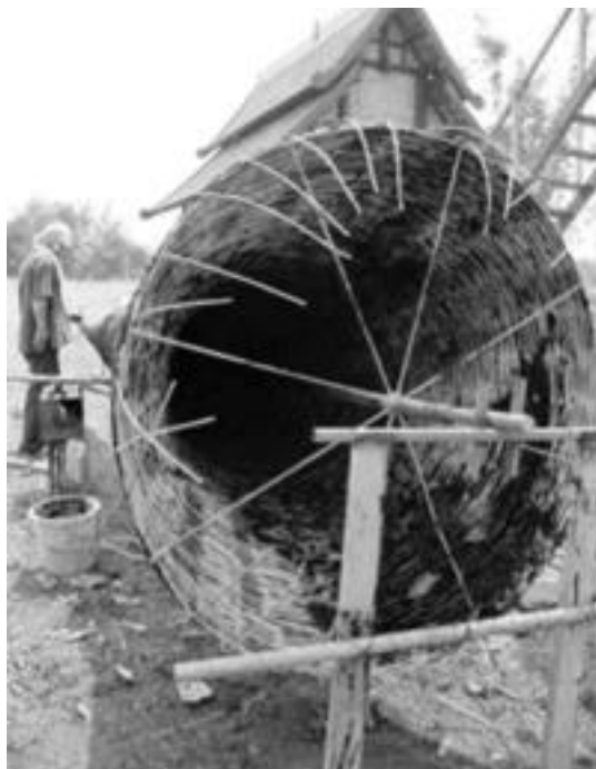
Figure 1. The image shows the upper section of the stupa still under construction. The bamboo strips are visible inside the structure (Photograph by researcher).
