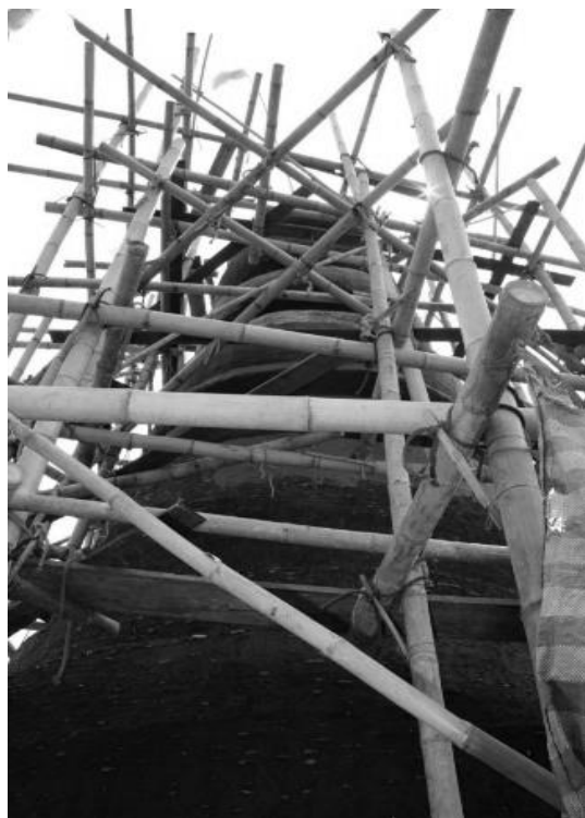
Figure 2. Bamboo stupa under construction. The image clearly shows the black lacquer and glue mixture on the surface of the bamboo stupa under construction. The lower part of the medhi is still lacking a final coat, so that the crisscrossed bamboo strips used to create the stupa as still visible (Photograph by researcher).
