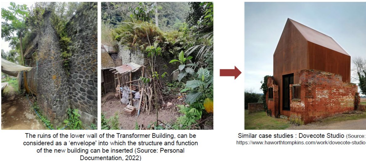
Figure 12. Utilization of the Transformer Building ruins by taking a case study of the insertion method in Dovecote Studio as a precedent
