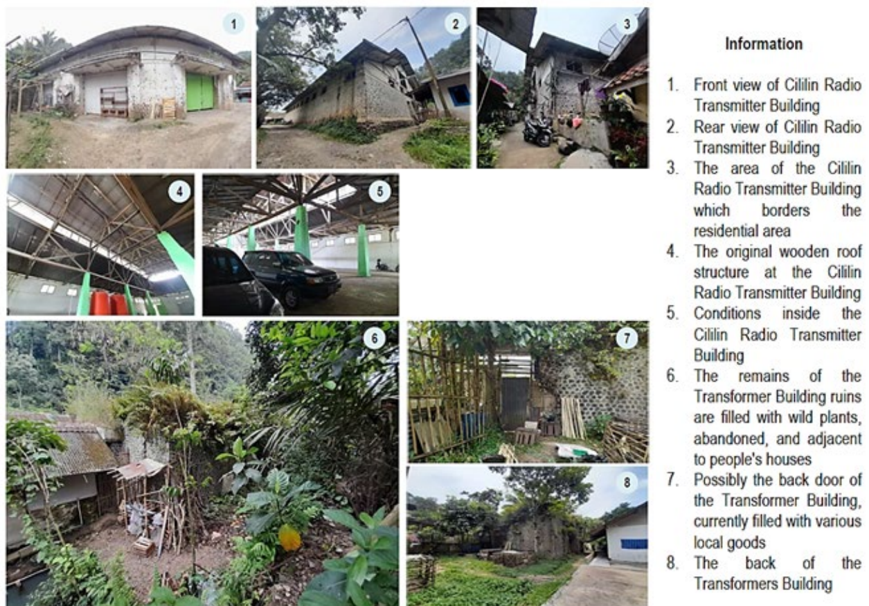
Figure 4. Existing Physical Condition of Cililin Radio Transmitter Building and Transformer Building
