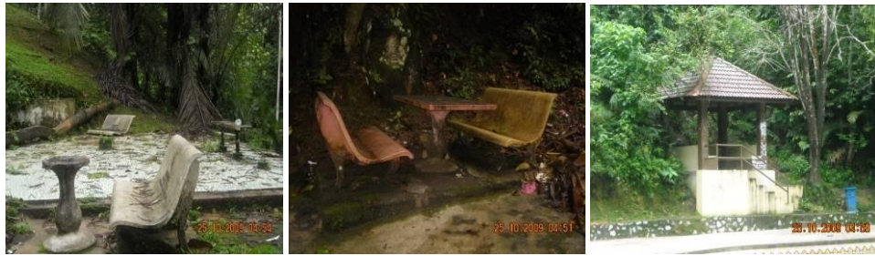
Figure 9: Some landscape elements in Templer Recreational Forest are unsafe to users and in bad conditions due to landscape maintenance system weaknesses, no inspection and lack of budget.
